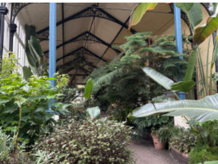
The Conservatory at the Pavilion Gardens in Buxton. A beautiful Victorian structure maintained by volunteers.
